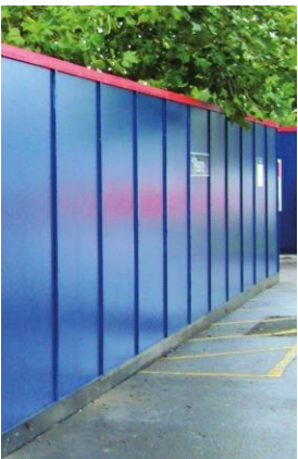
Example of Construction Site Boarding
